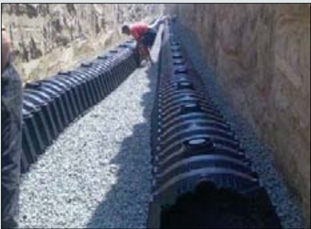
Infiltration system with GRAF infiltration tunnel, Galati (RO)
