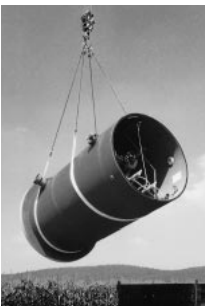
Unloading of the shaft with a crane
