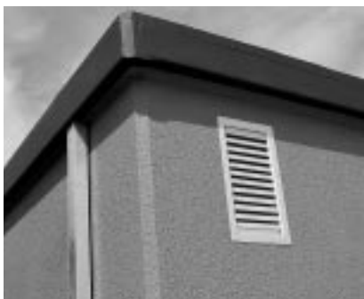
Down-pipes and ventilation grille in aluminium
