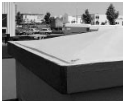
Shaped rain channel in roof
