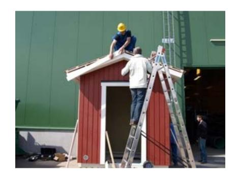
Last components to install will be roof sheets, battens and door.
