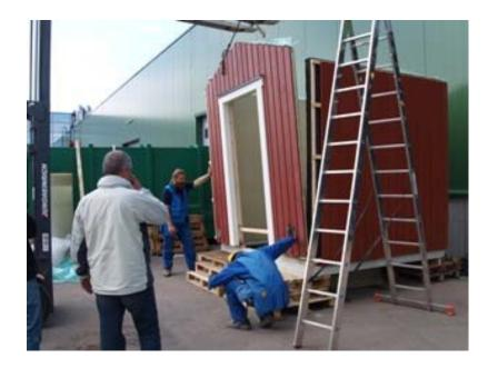
Panels will be lifted to their position and connected to fundament one by one.
